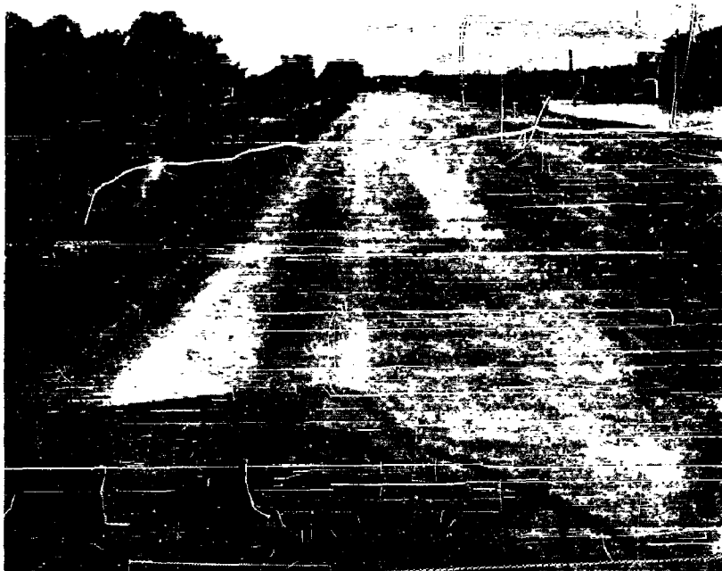
Speed-reducing wet season road deterioration.
